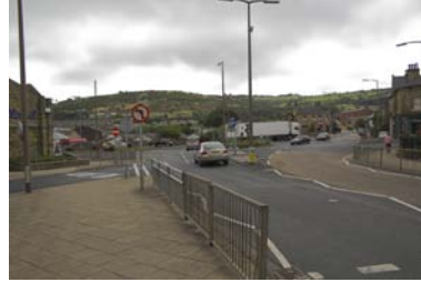
Picture 24 View southwards towards Elland Riorges Link roundabout.
