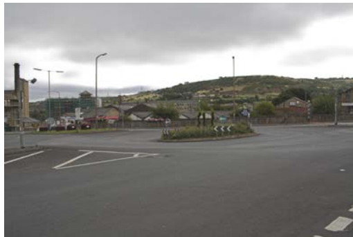
Picture 22 View of Elland Riorges Link roundabout
