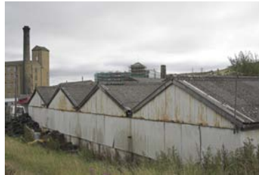
Picture 21 Low quality development off Dewsbury Road
