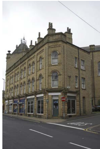
Picture 26 View of Town Hall rear elevation
