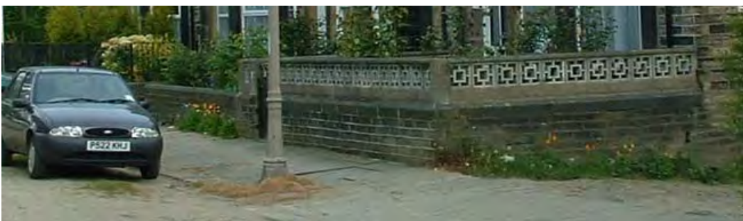
Boundary walls altered by adding concrete blocks
