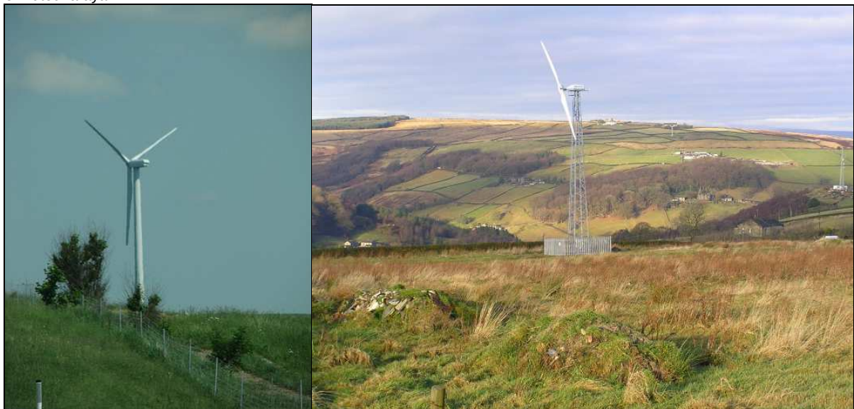
Typical three- and two-bladed turbines
