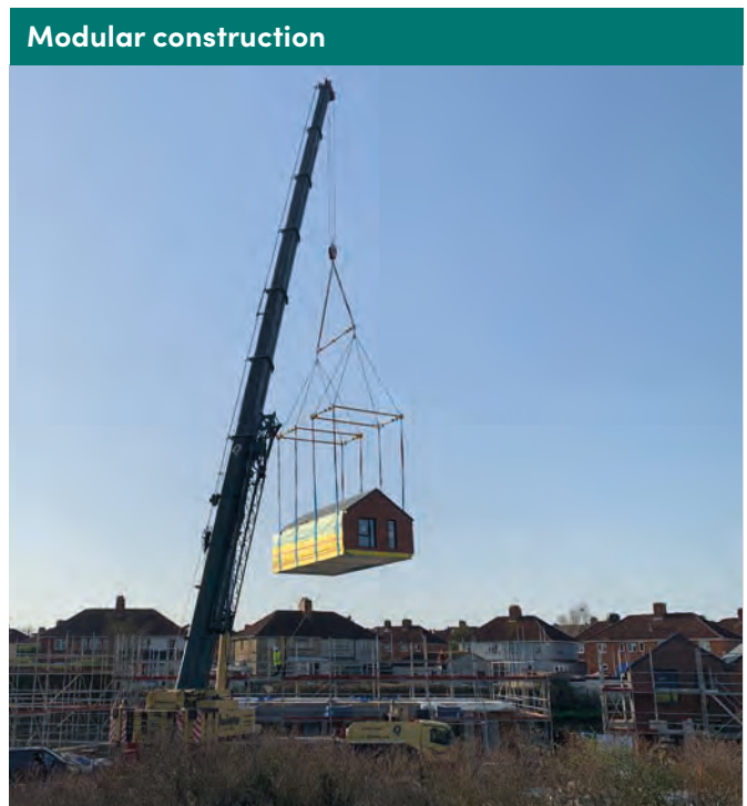
Housing modules manufactured off-site and quickly assembled on-site – Airport Road, Bristol.
