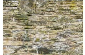
Local sandstone used for building and boundary walls, laid in a variety of bonds, with distinct variations in texture, shape and finish
