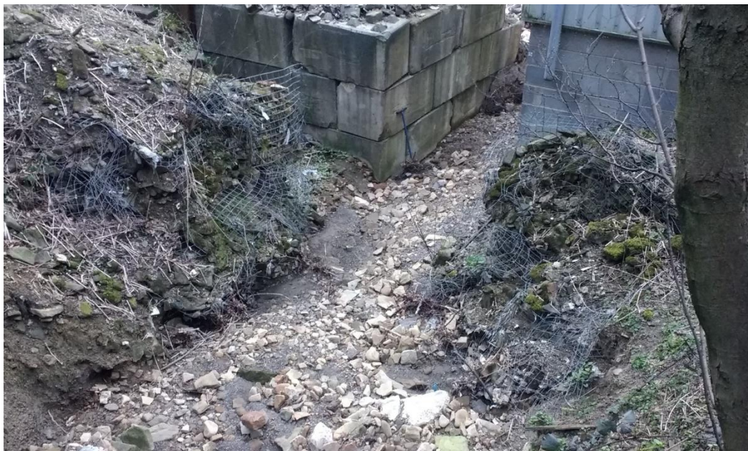
There is a pipe beneath this debris which would take the water under the rear yard from this area and exit into the River Ryburn
