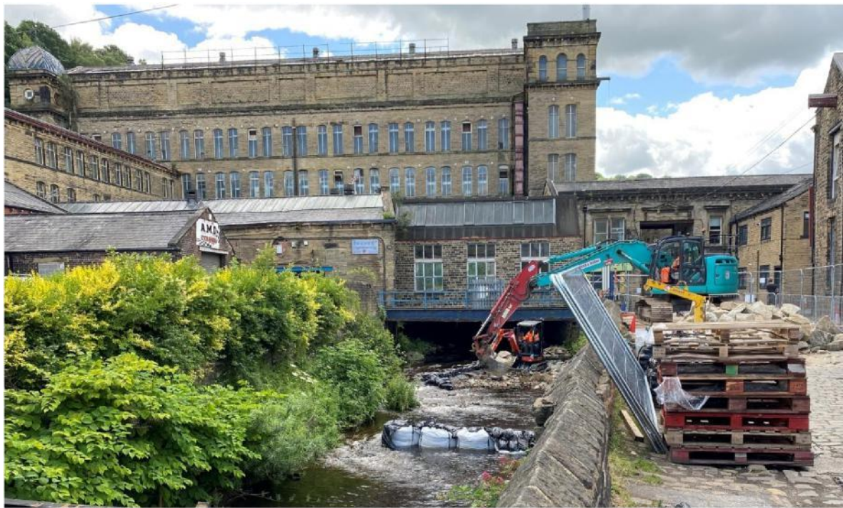
Work being carried out to install a fish pass on the River Ryburn in June 2023
